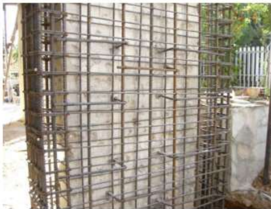
Fig. 3. Seismic upgrading with RC jacketing [Source: Courtesy C. Chrysostomou, TUC].
