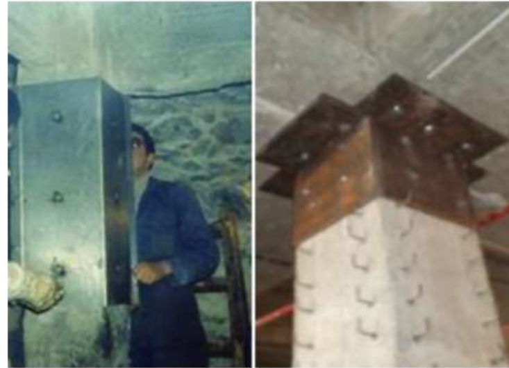
Fig. 4. Seismic upgrading with steel jacketing.
