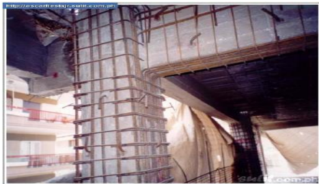
Fig: Concrete Jackting
