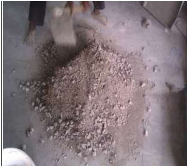
Fig : Initial Mixing of Constituents of Concrete
