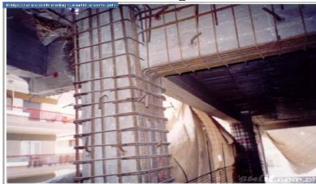
Fig: Concrete Jackting
